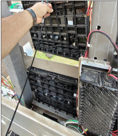
Figure 39: Pass Module Through Cutout
