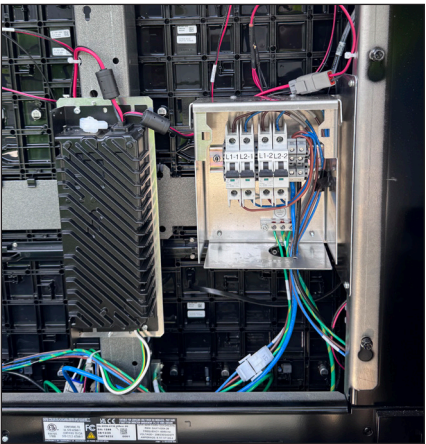
Figure 24: 40 A Termination Panel
