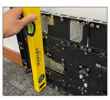
Figure 14: Ensure Panel Is Level & Vertically Flatness
