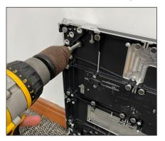
Figure 13: Secure Panel with Screws
