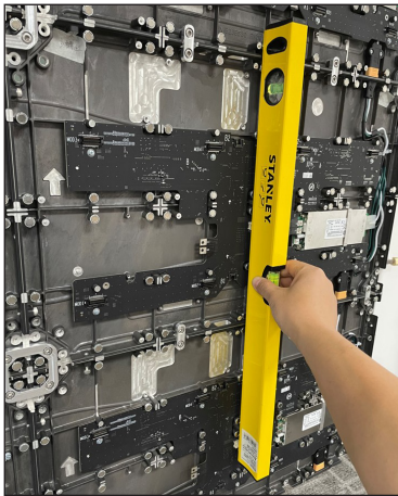
Figure 25: Verify Flatness with Level
