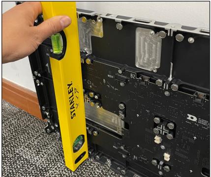
Figure 14: Ensure Panel Is Level & Vertically Flatness
