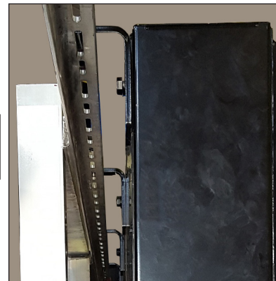
Figure 2: Clip Angle on Stringer
