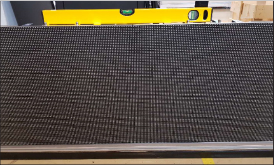
Figure 34: Ensure Panels Are Level & Plumb
