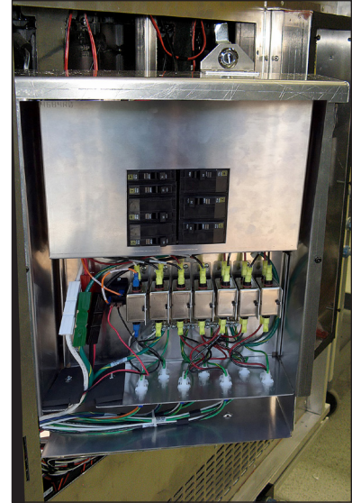
Figure 18: Swing Term Panel Out of Display
