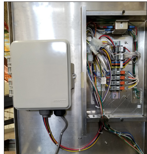
Figure 36: SmartLink™ Relay Bank
