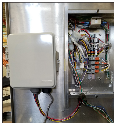
Figure 7: SmartLink™ Relay Bank
