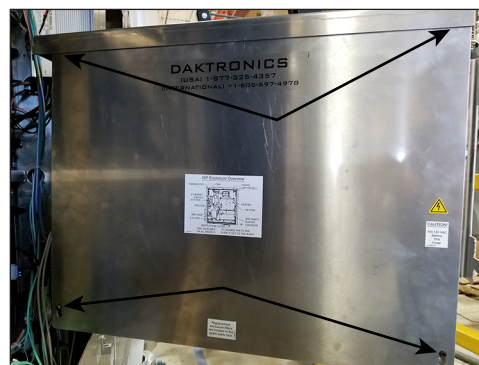
Figure 33: Control Equipment Door
