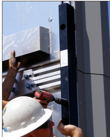
Figure 15: Aligning and Installing the Vertical Splice Tubes
