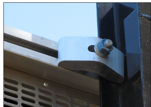
Figure 5: Rocker Clamp Engaging Upright
