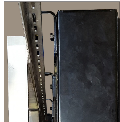
Figure 2: Clip Angle on Stringer
