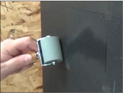
Figure 48: Roll at 45° Angle
