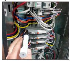
**4.** Remove K1 relay assembly by inserting the precision flathead screw driver on the release tab and leaning the screw driver toward the relay.
