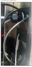
**11.** Disconnect the 3-pin mate n lok harness that is tied up above the second cable entry slit.
