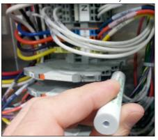
**5.** Remove the two spacers located above the K1 relay to allow room for the new relay.
