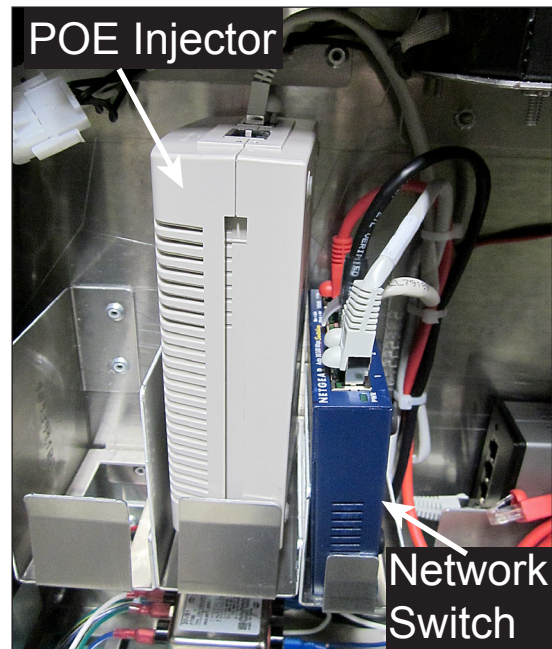
Figure 19: POE Injector and Network Switch in ISP Enclosure
