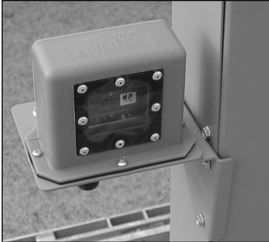
Figure 20: MDLS Installed Left of Display Face
