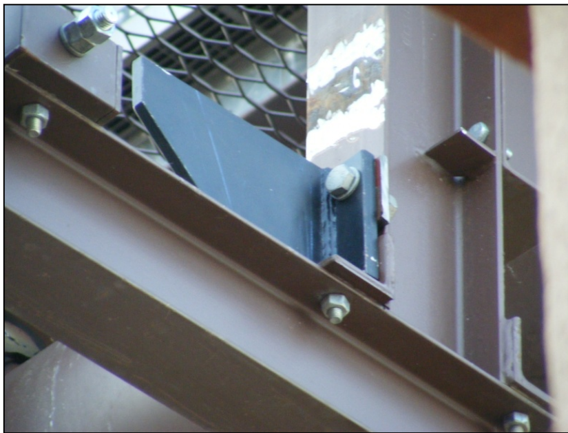
Figure 4: Installed Ledger Bracket
